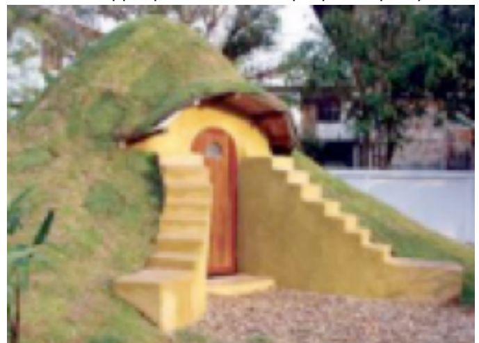
Necessarily exposed entrance to an "Earthbag" home http://earthbagplans.wordpress.com/introduction/
