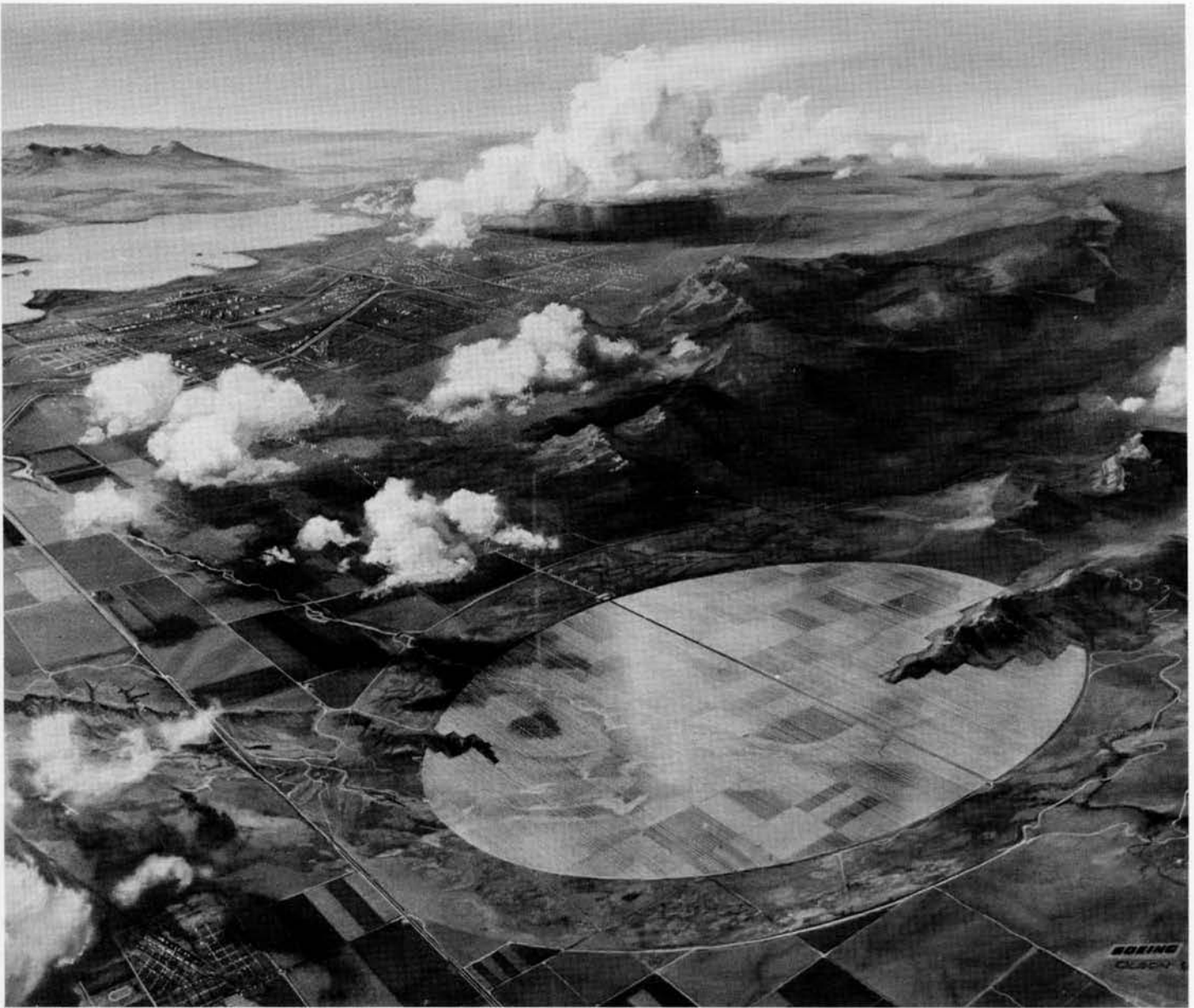
The microwave receiving rectifying antenna (rectenna). The uncultivated area around it has been closed to human access in order to limit microwave exposure. Under the rectenna the microwave level is very low, allowing cultivation of crops.
