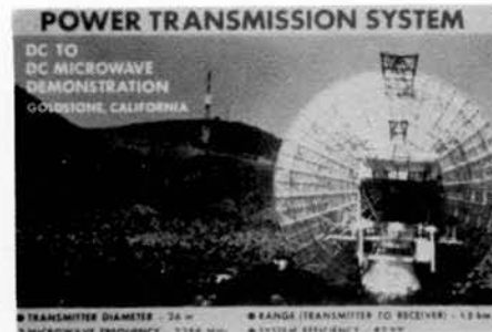
D23 Microwave power transmission test (summer of 1975).
