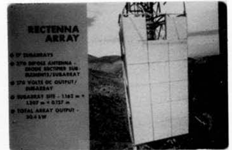
D24 Microwave power transmission test (summer of 1975).
